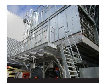
Designs for support dunnage steel, walkways, ladders and accessory supports (e.g., intake and discharge silencers)
