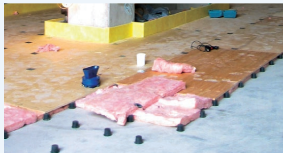
Floating floor installation for mechanical equipment room.
