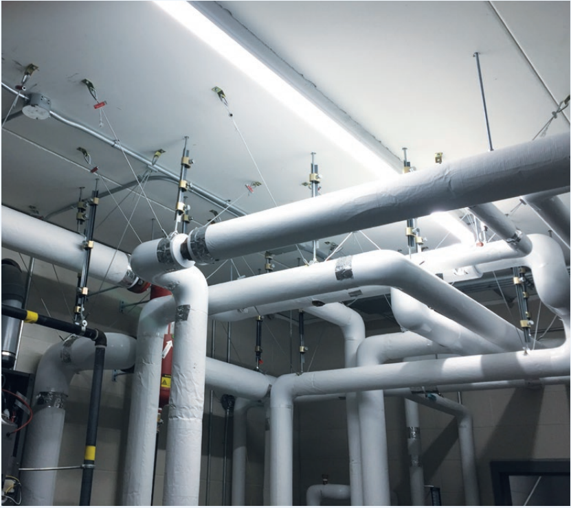
BulletBrace™ cable restraints, here installed on natural gas and heating water pipes, are quick and easy to install, taking just a few minutes per point. The rod stiffeners and clamps shown help ensure the threaded rods can withstand seismic uplift forces. These pipes are protected against damage from design-level earthquake events.
